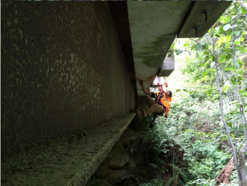
Photo #14 Girder 1 - looking to camp end
