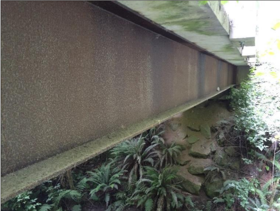
Photo #13 Girder 1 – looking to camp end
