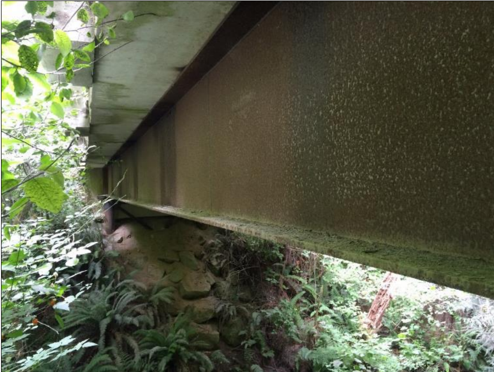
Photo #3 Girder 1, U.S, looking towards woods end
