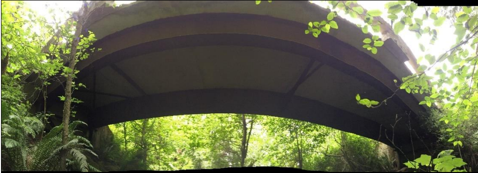
Photo #1 Downstream elevation / underside
