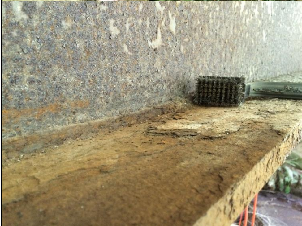
Photo #16 Girder 2 exterior / D.S face
